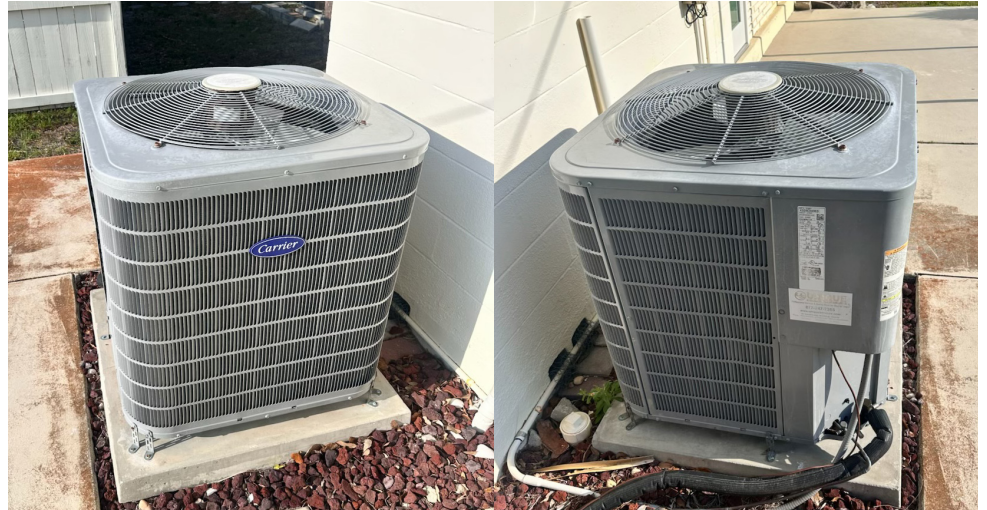
Coated with SIMIX Multi-Surface Ceramic Clearcoat. Installed Spring 2022.
