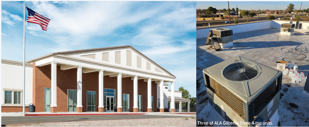
ALA Gilbert South Pre-K-6 Elementary School is located in Phoenix's East Valley area, Three of ALA Gilbert's Trane 4-ton units
